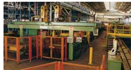
Heat treatment tunnel furnace
